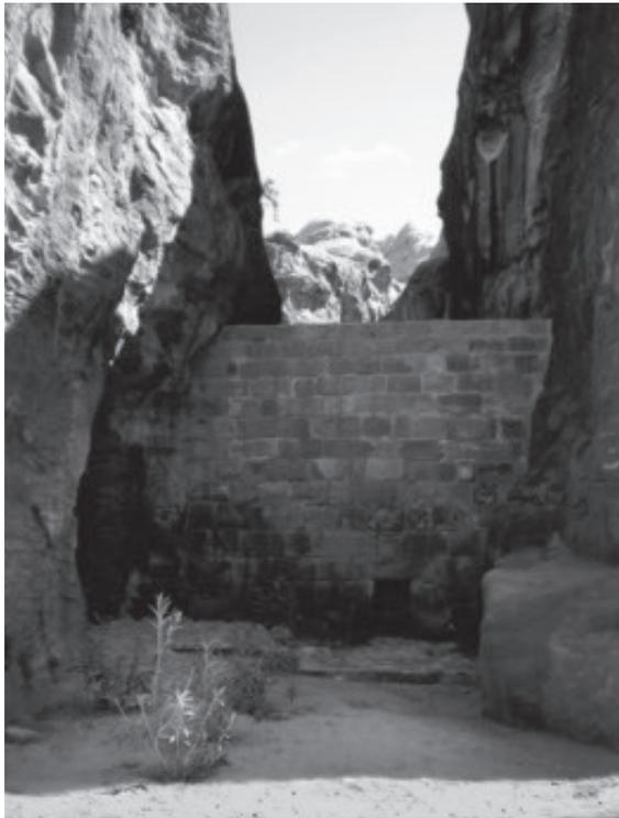
**Figure 4.** Dam at Petra to detain the impacts of flash floods. After Bagg (2012, 327 fig. 3).
